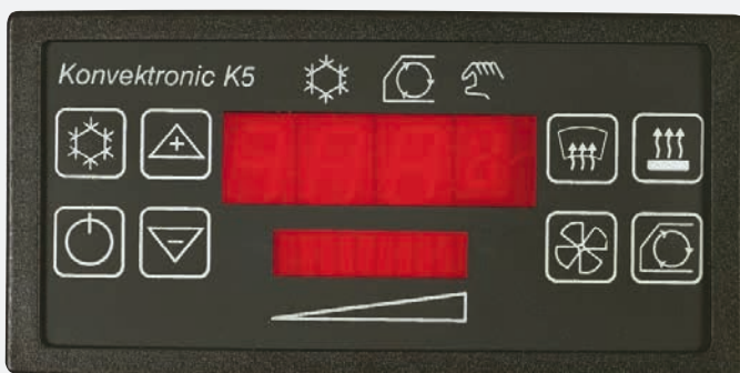
Air conditioning control panel.
