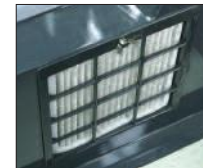
Recirculation air filter
